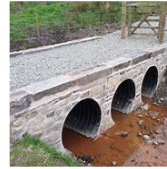
Bridges and Culverts $731,500
