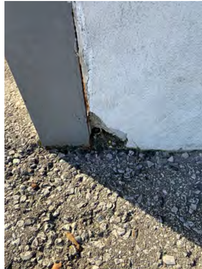
Photo 36 - South Elevation Opening
