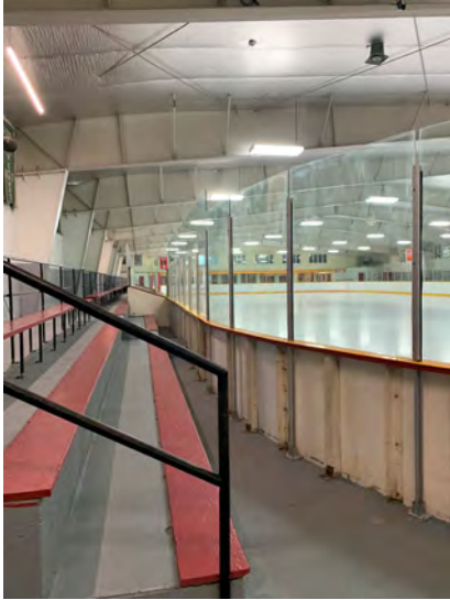
Photo 01 - Pre Engineered Frames
