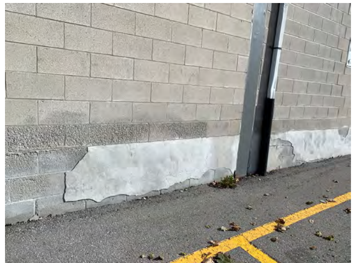
Photo 48 - North Elevation Parging
