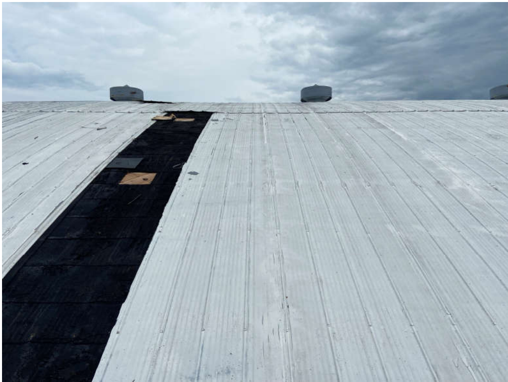
Photograph 10: Exposed roof deck at randomly selected location at west side of building
