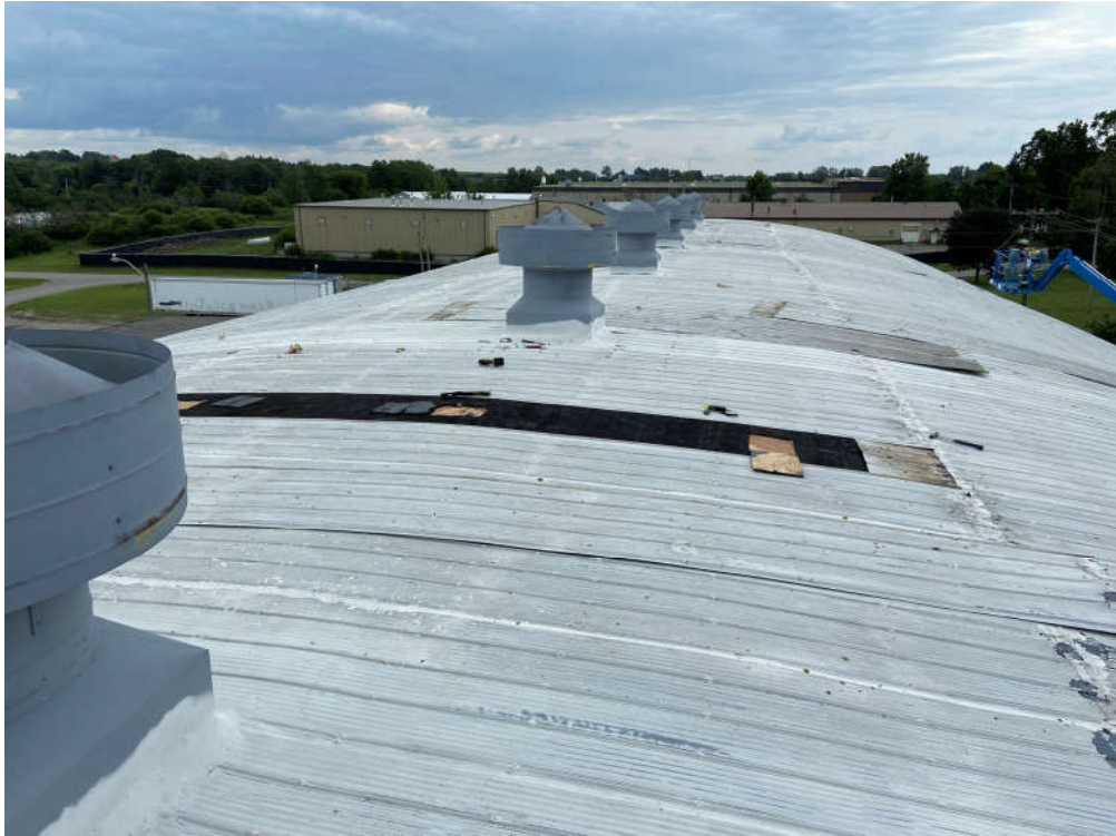
Photograph 11: Overview of exposed roof deck at randomly selected location at north end of building
