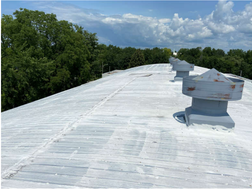
Photograph 7: Overview of existing metal roof
