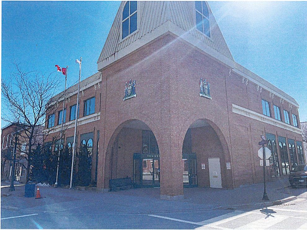
Photograph 3.1.8: Front Brick Arches
