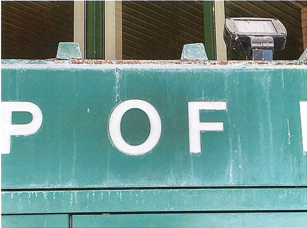
Photograph 3.1.2: Minor Corrosion
