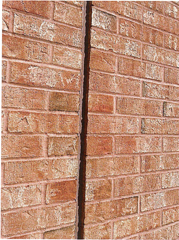
Photograph 3.1.13: Expansion Joint Seal
