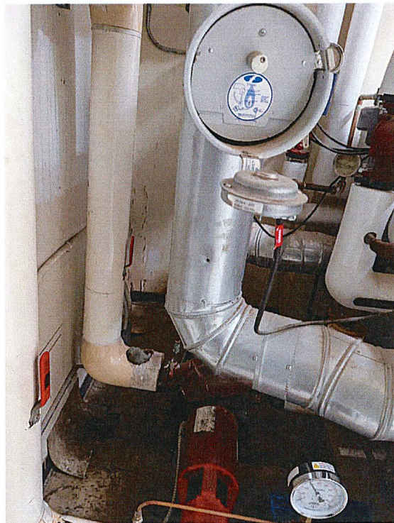
Photograph 3.2.1.3: Cable on Exhaust Duct
