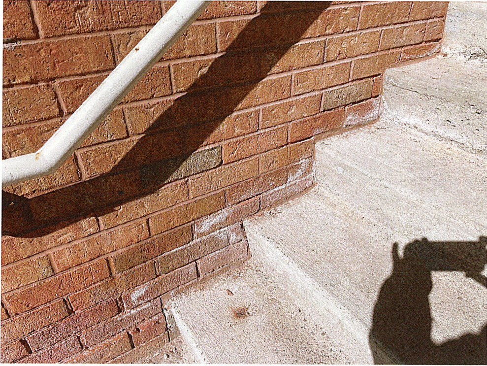
Photograph 3.1.12: Efflorescence
