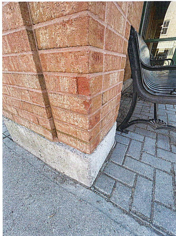
Photograph 3.1.11: Brick Repairs
