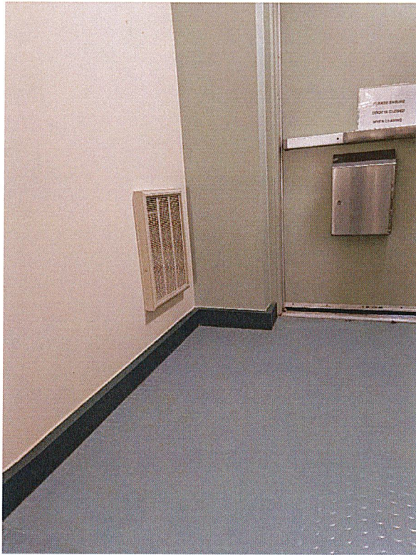
Photograph 3.3.4.3: Electric Heating
