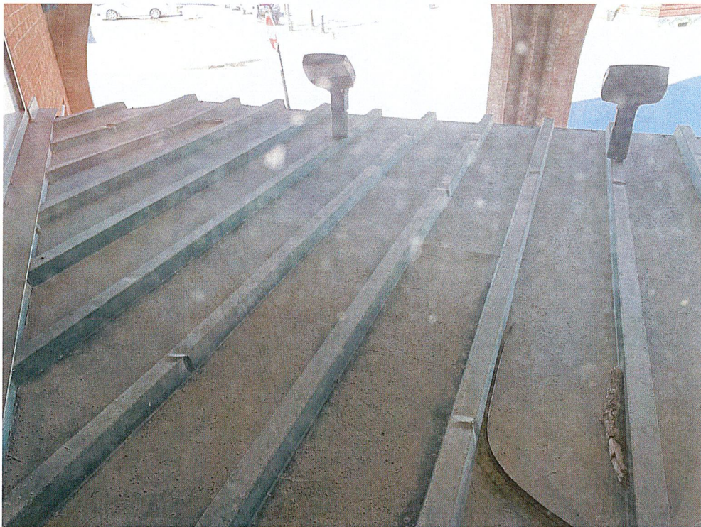
Photograph 3.1.4: Front Entrance Deck
