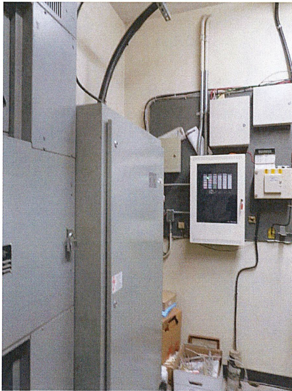
Photograph 3.3.1.2: Transfer Switch
