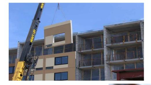
An example of an EIFS panel being installed where rasping may have been done in a controlled environment such as the factory where the panel was assembled.
