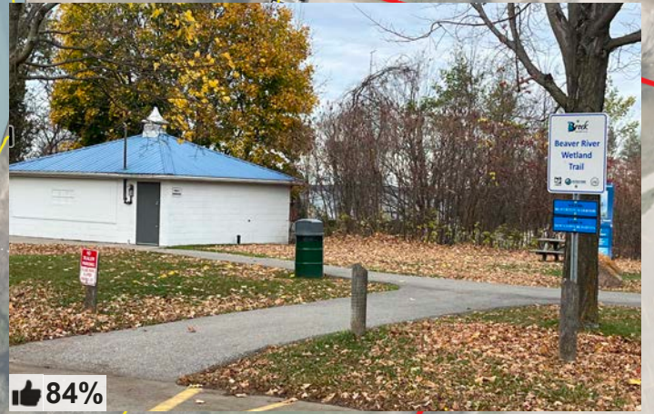
Washroom Upgrade washroom in its current location.
