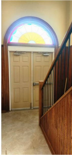
FIG. Div.8. 7 – East Exit Doors
