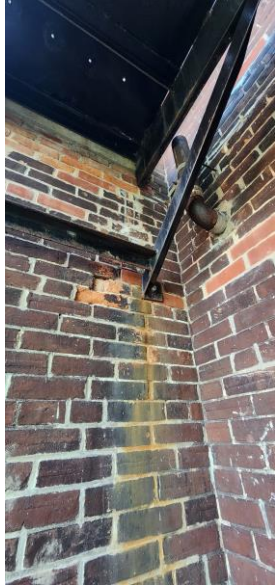
FIG. Div.5. 5- West Fire Escape Anchorage
