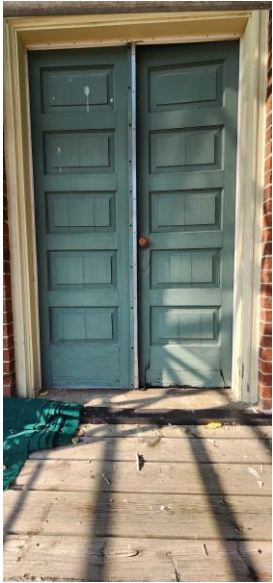
FIG. Div.8. 3 – Balcony Doors (Exterior)
