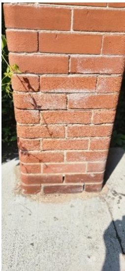
FIG. Div.4. 4 - West Entrance Canopy Column.
