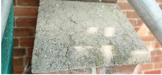
FIG. Div.3. 5 – Front Buttress Cap Stone 4
