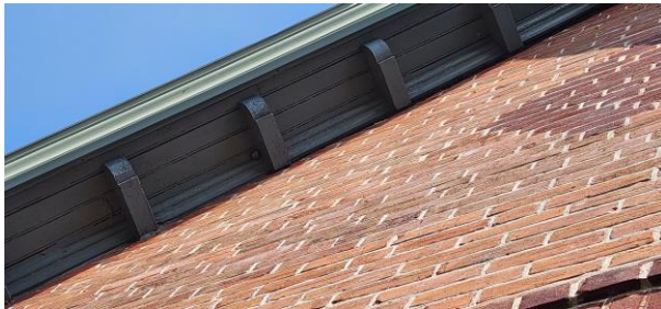
FIG. Div.6. 7 – Main Roof Painted Wood Soffit
