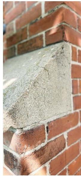
FIG. Div.3. 4 – Front Buttress Cap Stone 3
