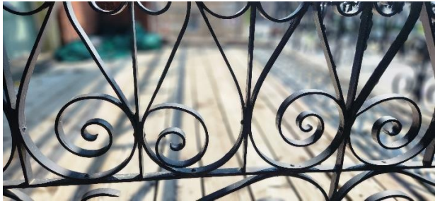
FIG. Div.5. 3 – Entrance Canopy Balcony Railing
