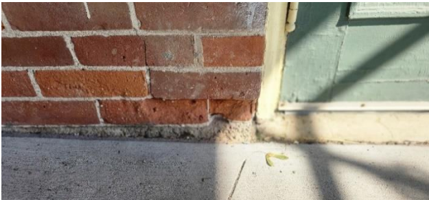
FIG. Div.4. 2 – Masonry at Exit Door
