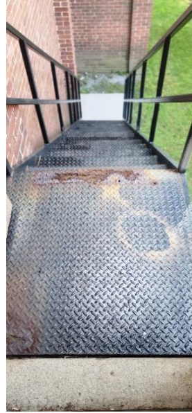
FIG. Div.5. 6- West Balcony Fire Escape Landing
