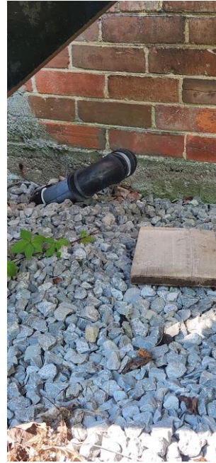
FIG. Div.15. 2– East Wall Projecting Vent Pipe
