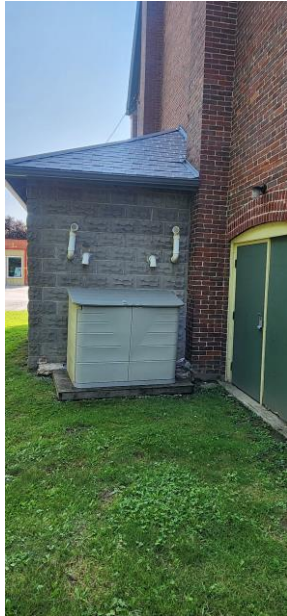
FIG. Div.15. 1 – Mechanical Room Addition
