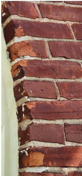
FIG. Div.4. 3 – Rose Window Masonry Surrounding
