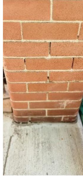
FIG. Div.4. 6– East Entrance Canopy Column
