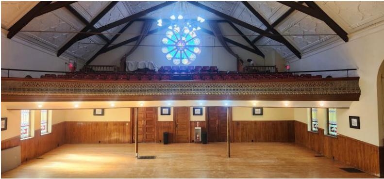
FIG. Div.1. 3–View of Auditorium From Stage
