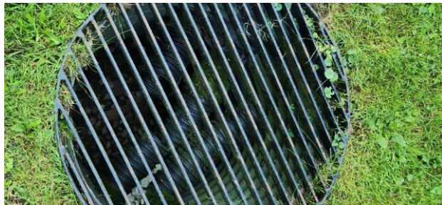
FIG. Div.2. 4 - Rear Area French Drain
