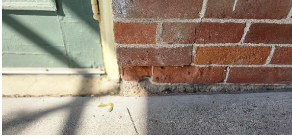
FIG. Div.4. 9 – Masonry at Exit Door
