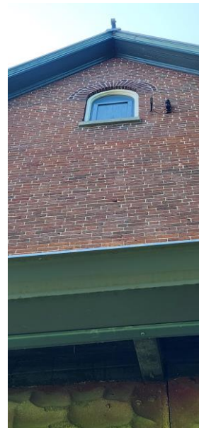
FIG. Div.8. 17 – Rear Elevation Attic Access
