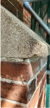
FIG. Div.3. 6 – Front Buttress Cap Stone 5
