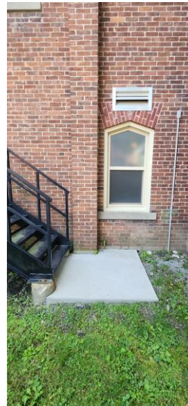
FIG. Div.8. 15 – Exposed Window at West Fire Escape
