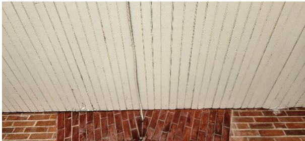
FIG. Div.6. 3 – Entrance Canopy Soffit
