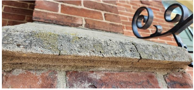
FIG. Div.3. 2 – Front Buttress Cap Stone.
