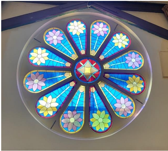
FIG. Div.8. 12 – Rose Window after Restoration.
