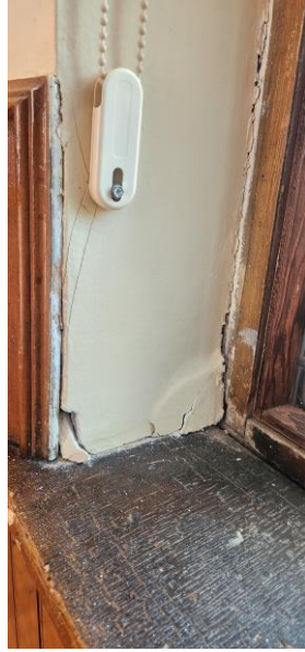
FIG. Div.9. 1 – Plaster at Auditorium West Window Sill
