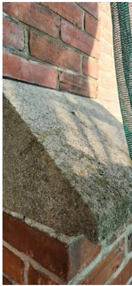
FIG. Div.3. 3 – Front Buttress Cap Stone 2
