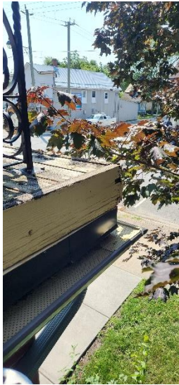
FIG. Div.6. 1 – Entrance Canopy Balcony Fascia
