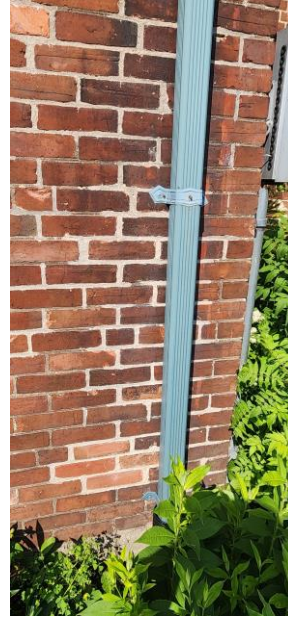
FIG. Div.4. 10– East Elevation Masonry at Downspout
