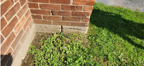
FIG. Div.3. 8 – East Wall Foundation
