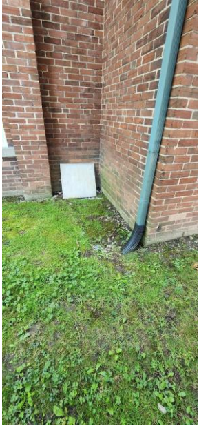
FIG. Div.7. 1- Buried Downspout Drainage
