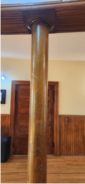
FIG. Div.5. 10 - Balcony Column
