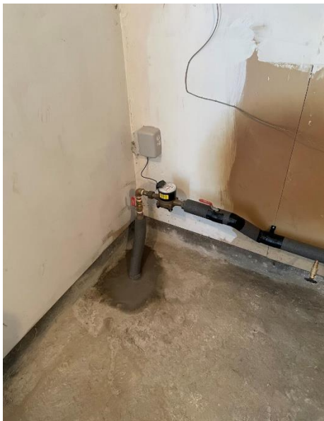
FIG. Div.15. 7 – New Water Line
