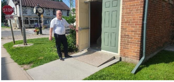
FIG. Div.8. 5 – East Exit Doors
