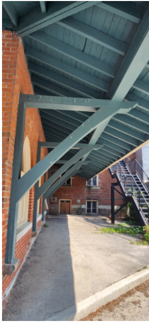
FIG. Div.6. 1 – View of Canopy at Service Ontario
