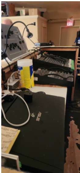
FIG. Div.16. 3 – View of Sound Board at Rear of Auditorium
