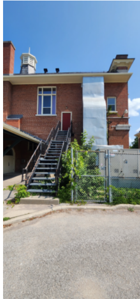
FIG. Div.15. 1 – View of West Façade at HVAC Unit
