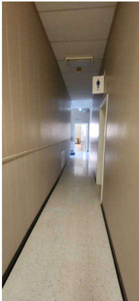
FIG. Div.9. 11 – Interior Exit Corridor with Painted Masonite Panelling 2
