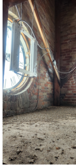
FIG. Div.4. 18 – Interior Clock Tower
