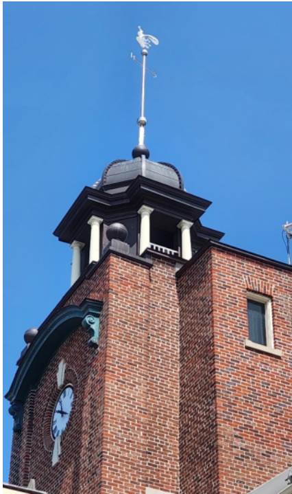
FIG. Div.7. 1 – View of Restored Tower Cupola
