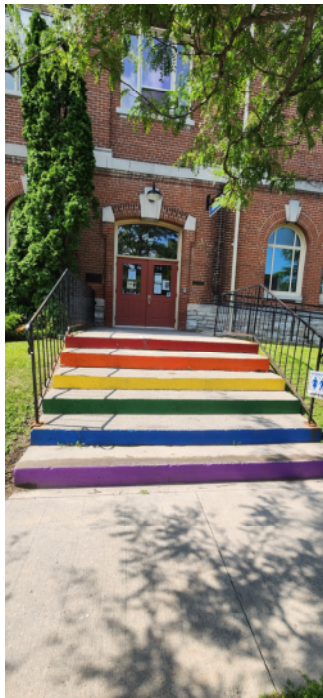
FIG. Div.2. 3 – Northeast Entrance
