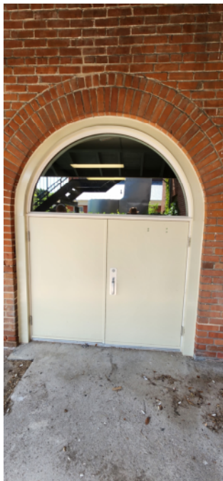
FIG. Div.8. 1 – Emergency Exit Door from Service Ontario (Exterior)
