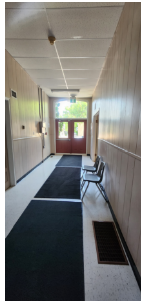
FIG. Div.9. 12 – Interior Exit Corridor with Painted Masonite Panelling 3
