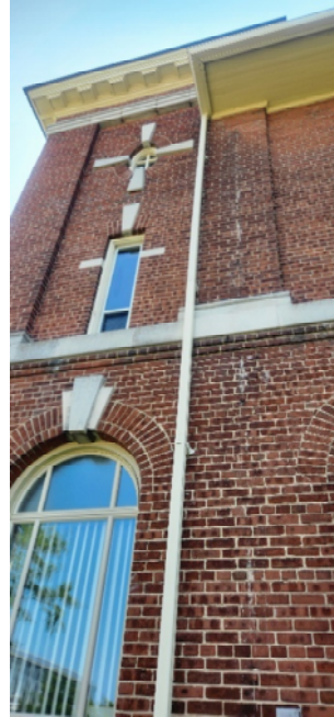
FIG. Div.4. 14 – North Facade
