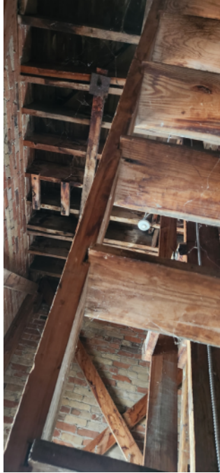
FIG. Div.6. 5 – Stair to Tower
