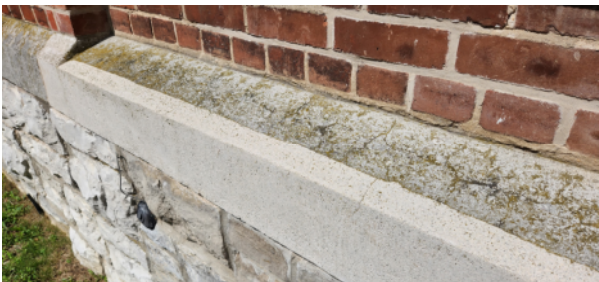
FIG. Div.3. 3 – Repaired Stone Sill
