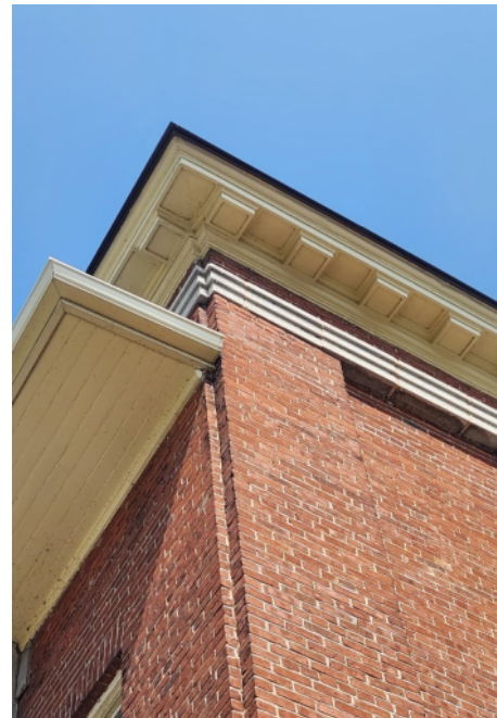
FIG. Div.6. 4 – Painted Wood Soffit
