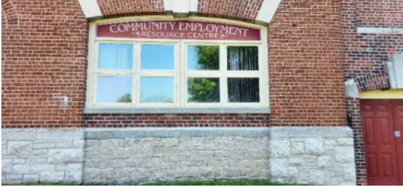
FIG. Div.8. 5 – North Façade at Old Doors Now Infilled
