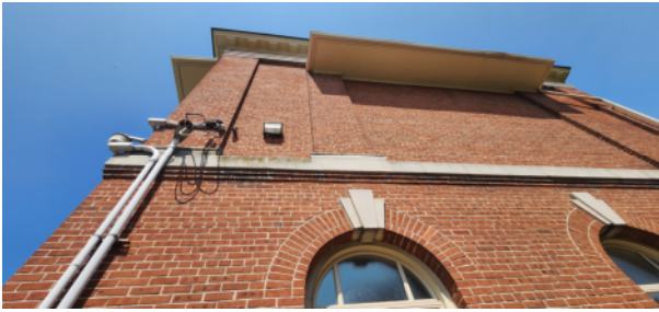
FIG. Div.4. 13 – General View of Tower Masonry
