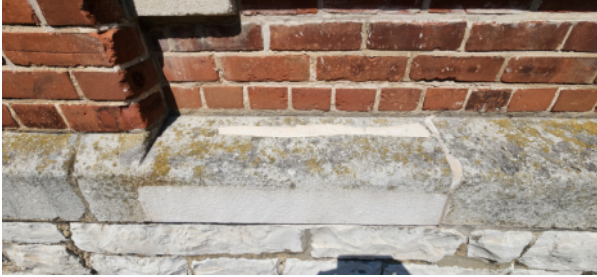
FIG. Div.3. 5 – Stone Sill Repairs
