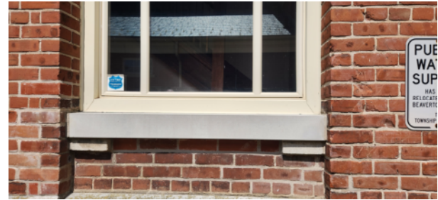
FIG. Div.3. 2 – Precast Concrete Sill Replacement
