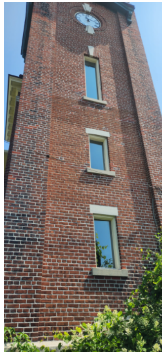
FIG. Div.4. 16 – General View of Tower West Façade 2
