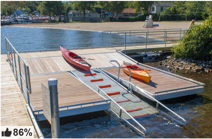
Canoe and Kayak Launch Add canoe and kayak launch (blue asterisk on the drawing on page 2) along the river on the land parcel on the south side of the railway.
