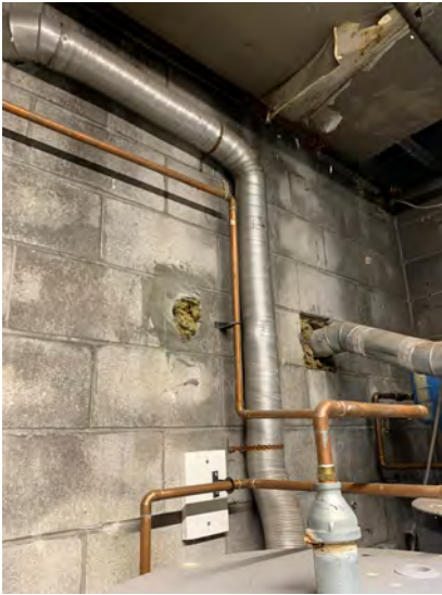
Photo 23 - Masonry Block Wall Efflorescence
