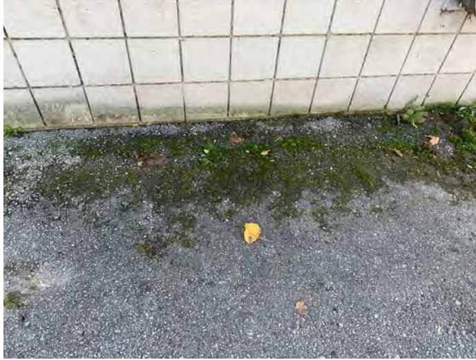
Photo 41 - East Elevation Vegetation
