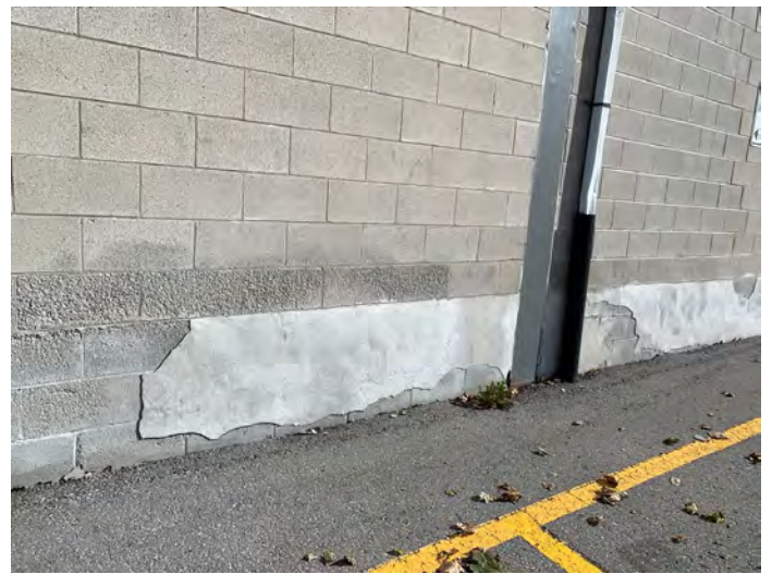
Photo 48 - North Elevation Parging
