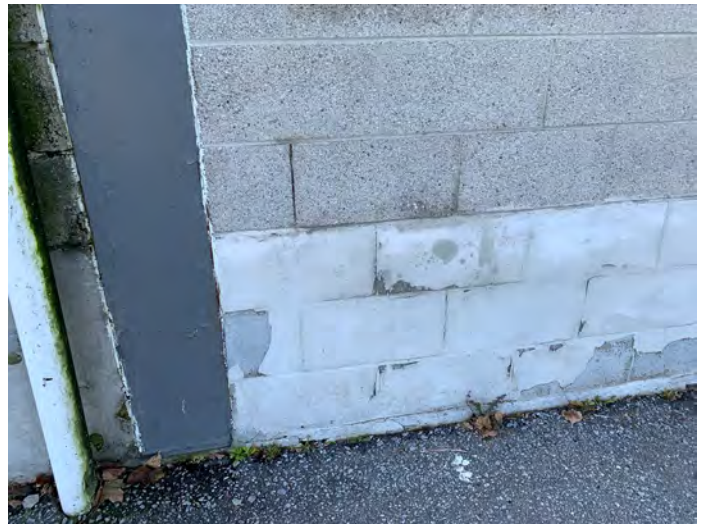
Photo 040 - South Elevation Block Wall Parging
