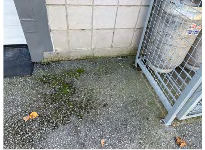
Photo 42 - East Elevation Vegetation 2
