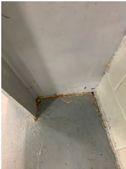
Photo 11 - Pre Engineered Frame Base Corrosion
