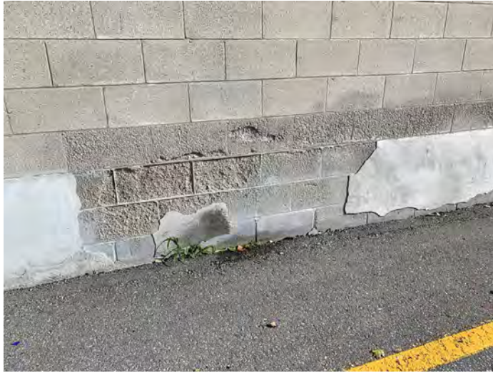
Photo 49 - North Elevation Parging2
