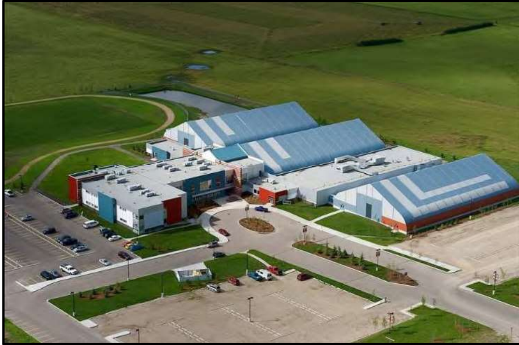
Picture 4 - Example of a multi-pad facility incorporating fibre membrane construction
