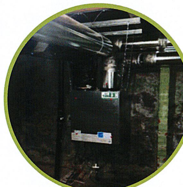
Energy recovery ventilator unit
